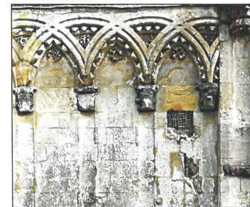
Fig. 42 Interlaced chevron mouldings in the Lady Chapel. The chapel shows evidence of the transition from Norman decoration to early English Gothic.
