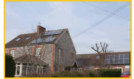
The package array below is based on a slightly off-South facing roof and has 10 panels. It is a 3.7kw system and the price of £3,968.13 includes all of the equipment and installation.
